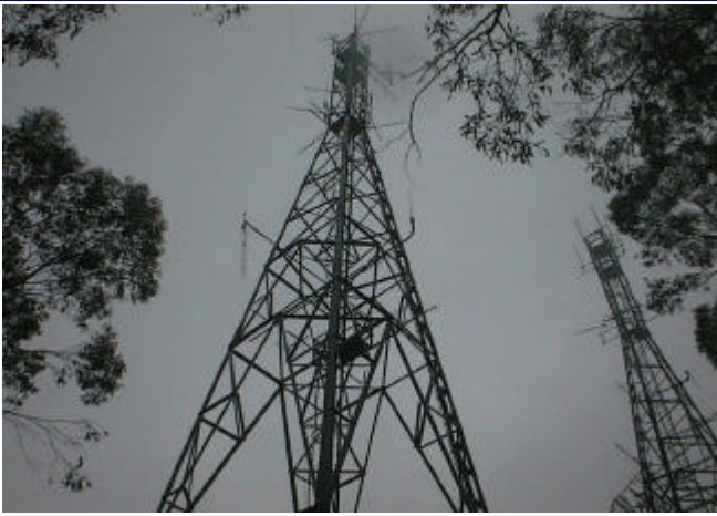
The Antenna Towers in the Clouds.
