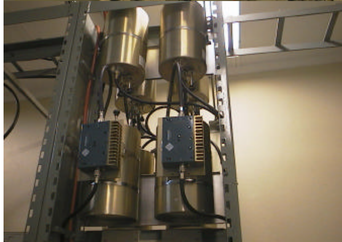
These two shots are of the Police UHF cavities just installed front and rear.
