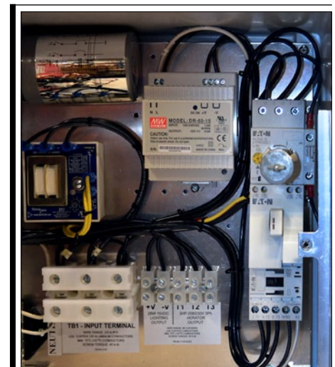
Fig. 7 | DC Power Supply/LED Light Controls mounted in PCC with a 3HP 230V/3Ph unit with Phase Monitor.
