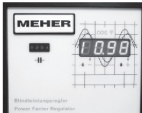
Relay indicating 0.98 lag power factor
