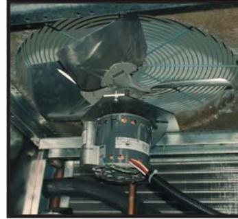
Typical fan assembly Figure 2.4A
