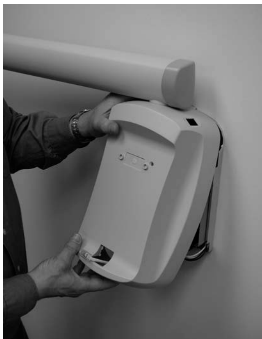
Figure 36 Placing the Cover on the Control Unit
