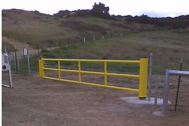
New gate at Blackstar Canyon site
