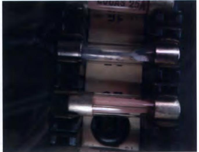
Any overheating that does occur, first softens the plastic that secures the fuse holders, causing the blades to open out and make even less contact with the fuses. This exacerbates the problem.
