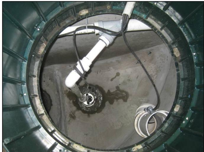
**IMPORTANT:** Do not lower the pump via the electrical cord.
