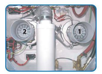
The vacuum motors are wired to two separate switches number one is wired to a loom and number two is wired directly to the number two switch. Below are four steps for easy vac motor replacement. Make sure if you replace a vac motor to remember to put back the piece of PVC around the vac motor's head. This is very important to have because it protects wiring in case any water ever passes through a vac motor.
