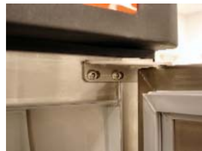
Right-side mounted upper refrigerator door hinge.
