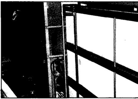
Damper plate and operating mechanism.
