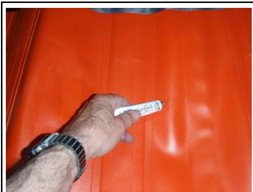
*Squeeze glue around the tear and spread with fingers.*
