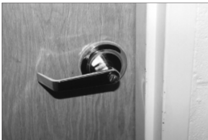
10. The inside rose and lever handle installed.
