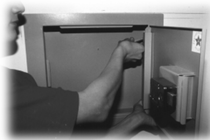
4. Place the safe in the cut out and mark the mounting screw holes.
