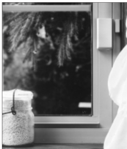
3. Door/Window sensors send an alarm signal to the control panel when their battery-powered circuits are broken. The small unit is a magnet; the larger unit contains the battery and radio transmitter.
