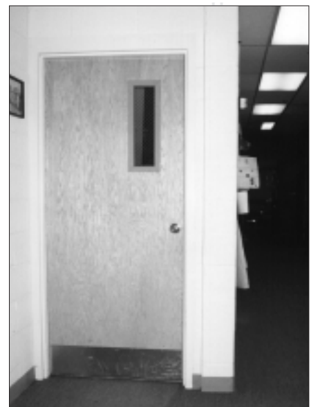
2. This and several other doors on this local business required lever conversion.
