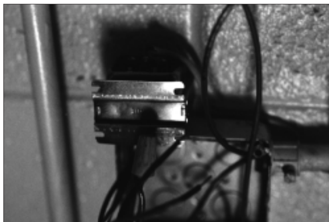
12. The Trine 125 transformer was hardwired to prevent accidental unplugging.
