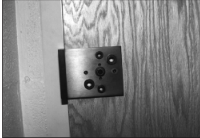
4. Place the HIT-1 guide over the crossbore.
