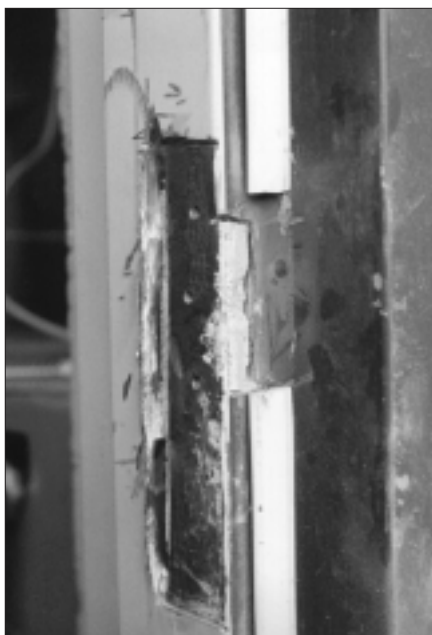
4. There's more to this door than jamb and mortar. Notice the thick steel plate found directly below the jamb.
