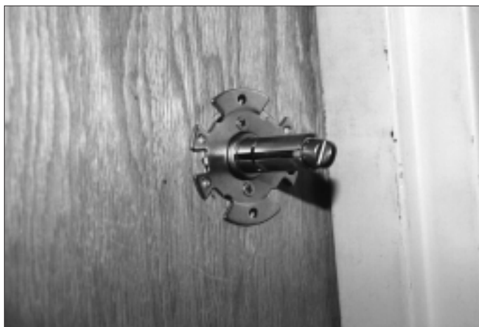
8. The lock housing and back plate are installed.
