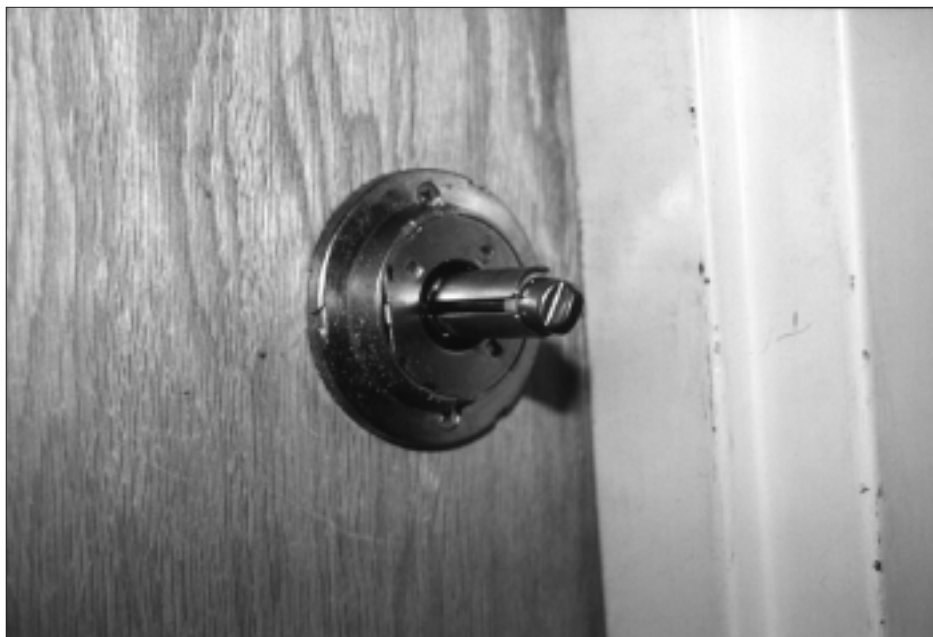
9. Inside spring cage attached.
