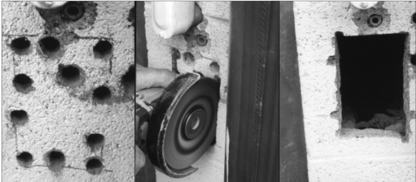
6. The mounting hole for the switch box is sketched, drilled and cut, making a perfect hole for placement.
