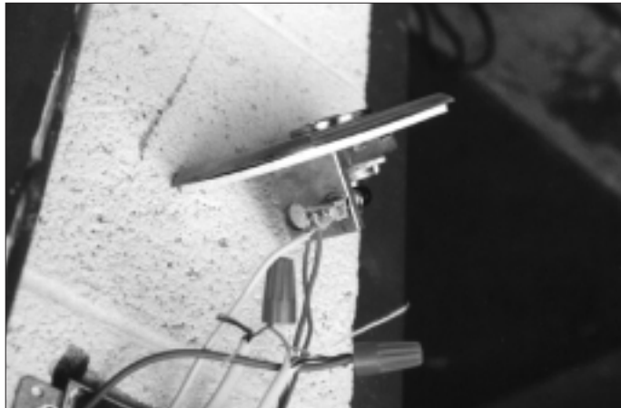
10. One switch wired and ready to go.
