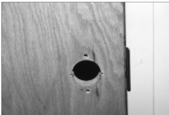
7. Door with completed support post and locator tab holes drilled.
