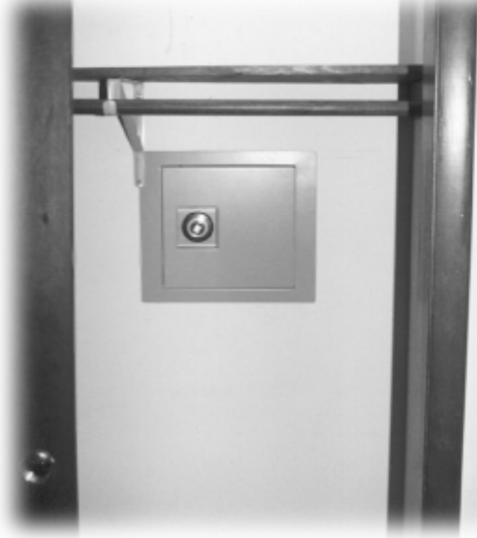
7. The completed installation: Door swings free and easy; door in closed position; the closet shelf and rod are replaced.
