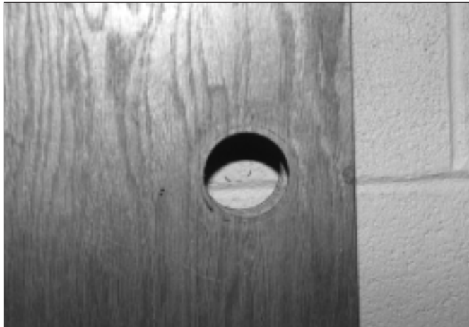
3. Drill edge and crossbore holes.
