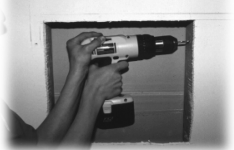
5. Use a 3/16" drill bit to drill pilot holes for the mounting screws.
