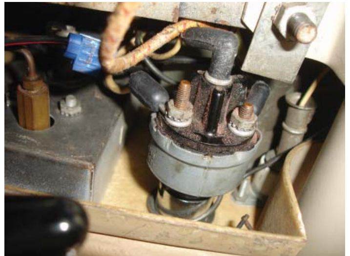
Here is the back of the ignition switch-. Notice the live terminals and their close proximity to the grounded steel z-bar. In last month's issue we showed you how to insulate this trouble spot using a simple aerosol can lid.
