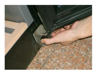
b.The bottom Hinge is fixed with four bolts, you should use a M6 sleeve to unfix it,
