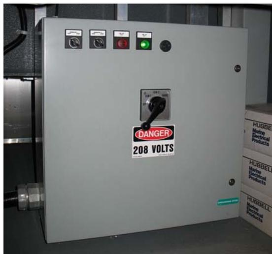
**Figure 19: 208V Power Control Panel**
