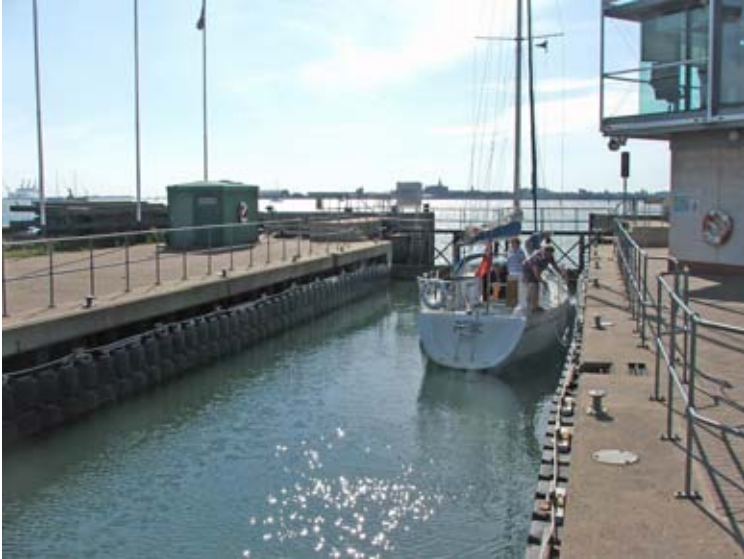
Shotley Marina lock with floating fenders and cleats.
