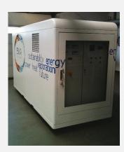
The unused steam is converted into carbon-neutral electricity which can be fed into the grid (CHP electricity) or can also reduce the own power consumption.
