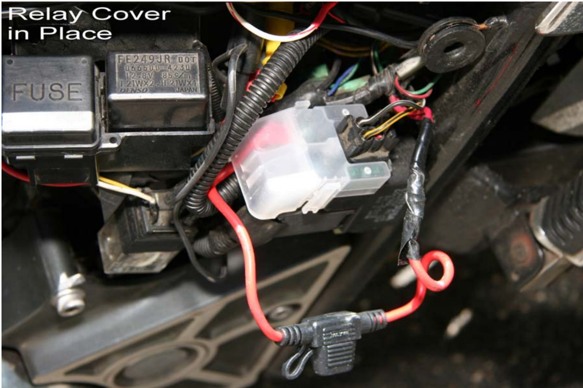
Starter Relay Cover in Place Showing Routing of Fuse Lead
