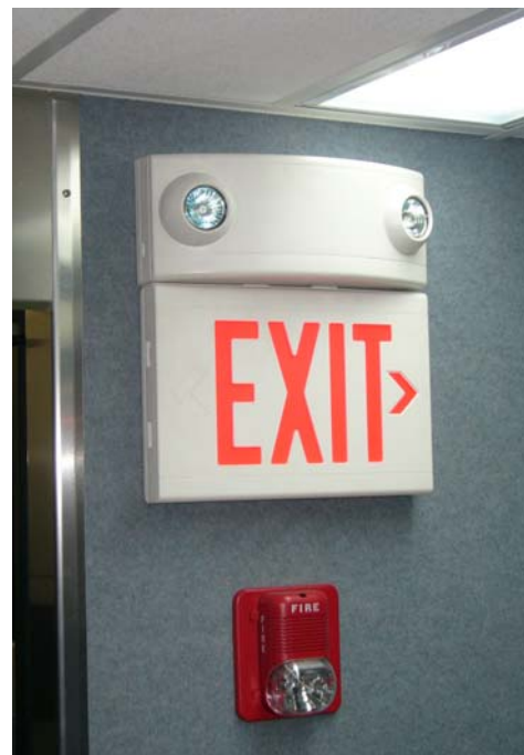
Figure 2: Emergency Lighting (Typical)
