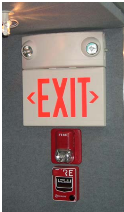
Figure 2: Emergency Lighting (Typical)
