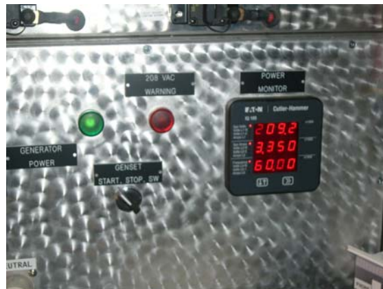
Figure 29: 208V AC Phase Power Monitors
