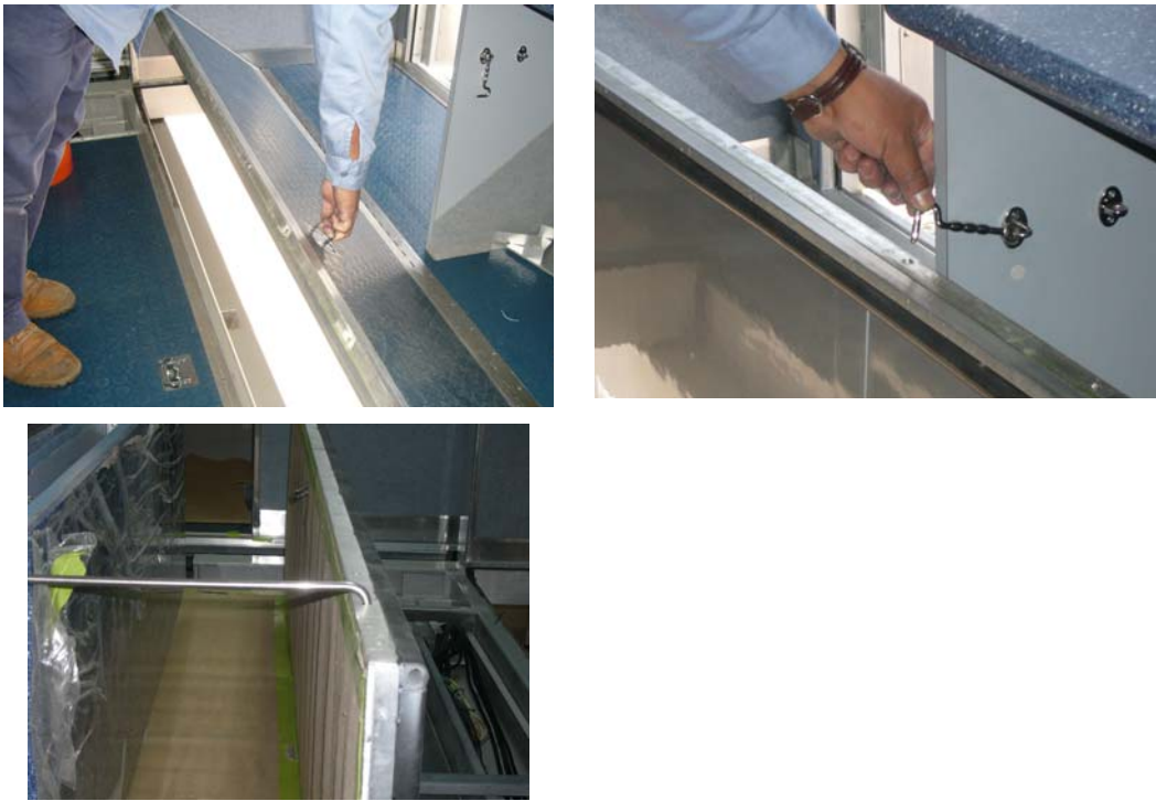
Figure 25: Securing Expando Floors
