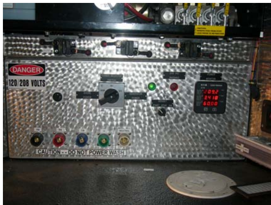
Figure 29: 208V AC Phase Power Monitors
