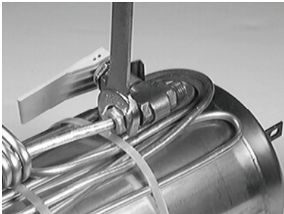
Figure 20: Vent Tube Removal
