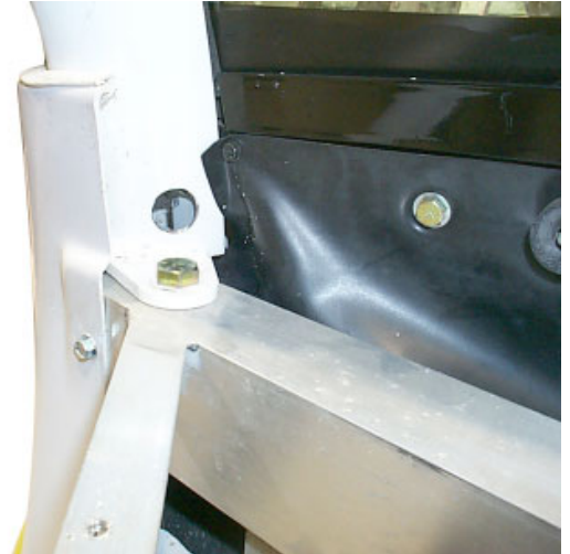
Fig. # 12 Drill lower hole in roof rail
