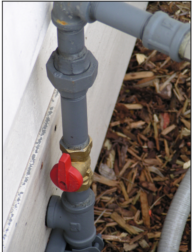
Figure 3-7 Manual Fuel Shut-Off Valve (outdoor installation shown)
