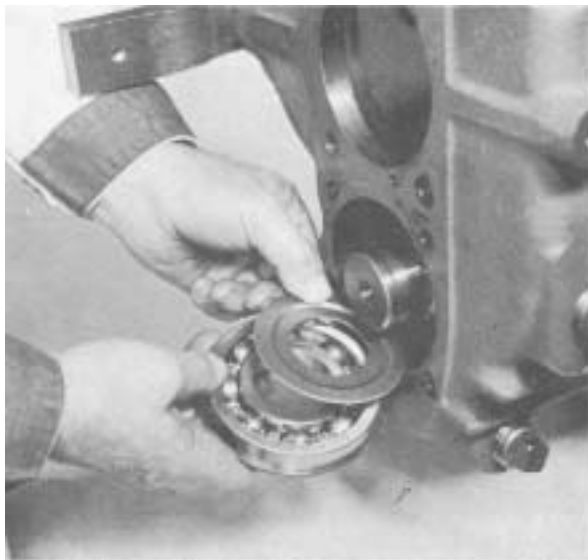
Figure 62 - Position rear bearing oil slinger as shown and start rear bearing.
