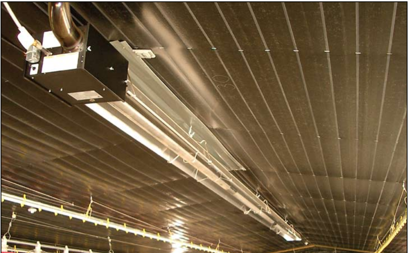
Gas-Fired, Low-Intensity infrared heaters heating a poultry house in the United States.
