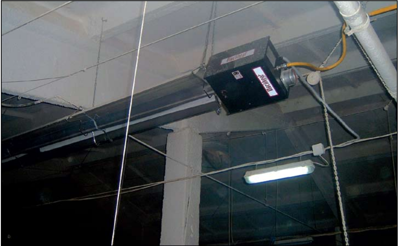
Gas-fired, low-intensity infrared heater being installed in a poultry house in Russia.
