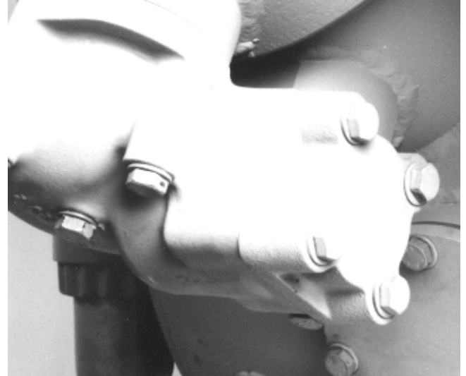
Fig. 2.3-1 Back pressure dependent relief valve
