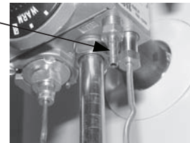
Pressure Tap Shown Installed
