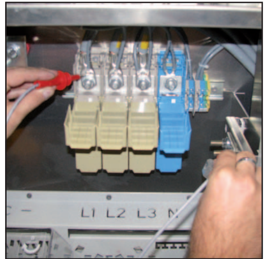
Example: Measuring the insulation resistance (PE to L1)
