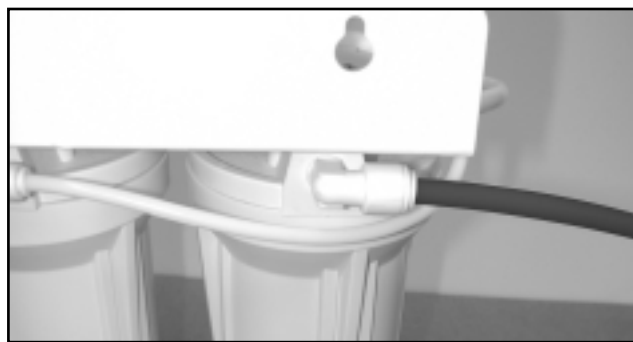
Figure 8 - Installing membrane without touching
