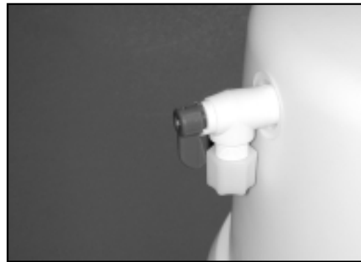
Figure 6 - Pressure Tank Shutoff Valve
