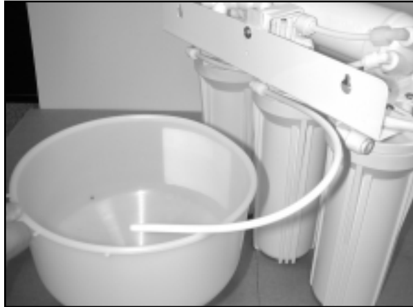
Figure 10 - Direct flushed water and carbon fines into container
