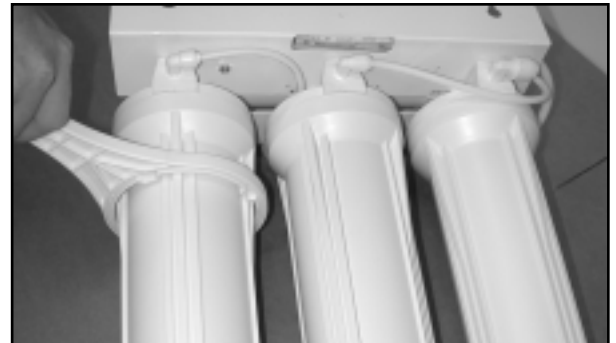
Figure 11 - Using sump wrench to change filter cartridges
