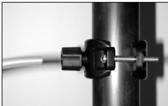
Figure 4 - Drain Saddle Assembly
