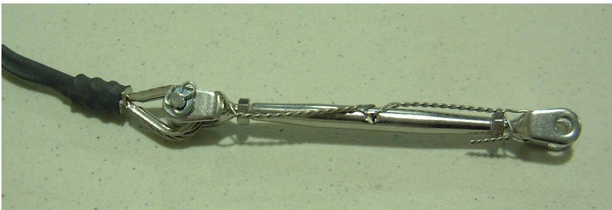
Acceptable wire locking of turnbuckle
