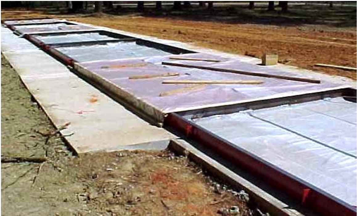
The scale assembly is ready to pour.
