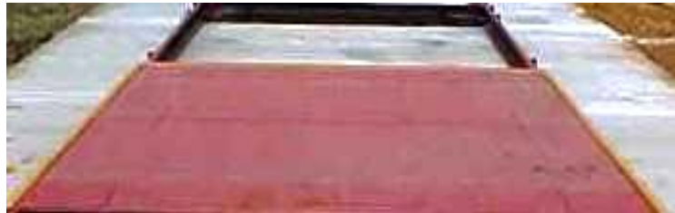
Place the Drive Axle Scale against the first Concrete Dead Space Frame .
