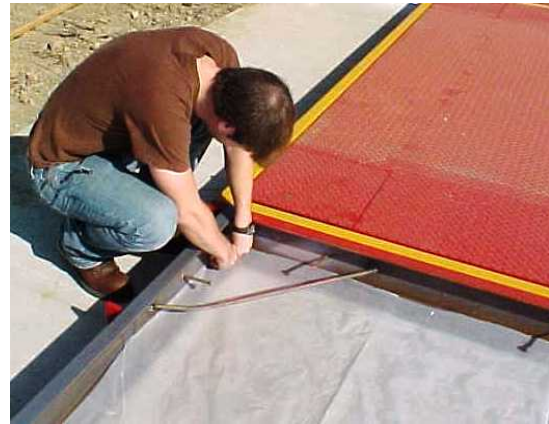
Tape plastic sheets to the inside of the frame.
