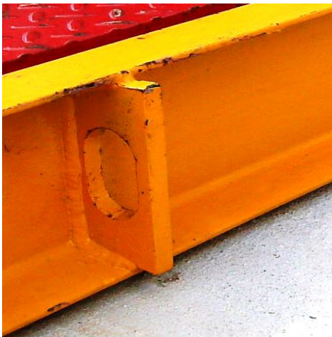
Scale and frame lifting points
