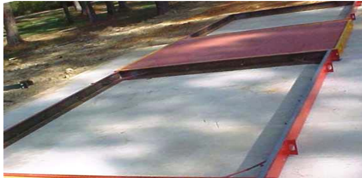
Place the Concrete Dead Space Frame against the Steering Axle Scale .
