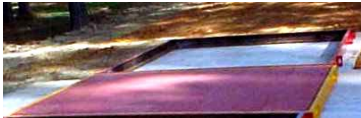
Place the Steering Axle Scale adjacent to the Approach Concrete Frame .
