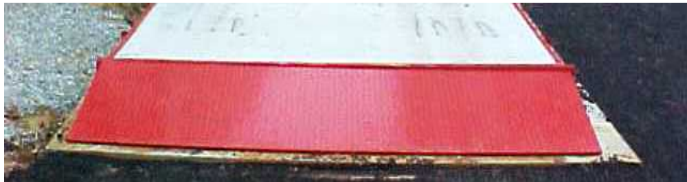
Bolt the Ramps to the Approaches
