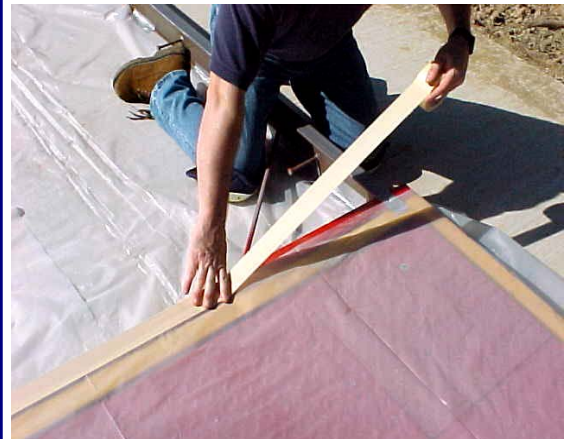
Cover decks with plastic.
