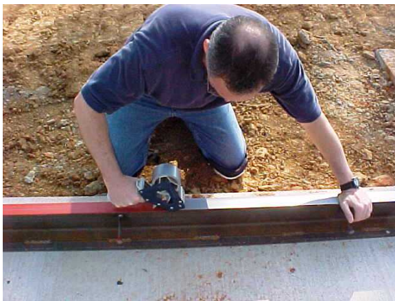
Tape edges of the concrete frame.
