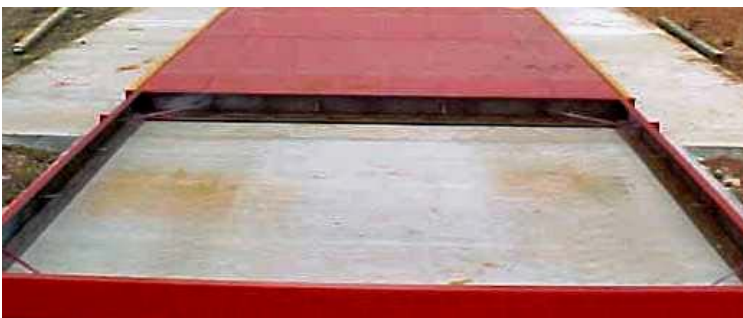
Place the Concrete Dead Space Frame against the Drive Axle Scale .
