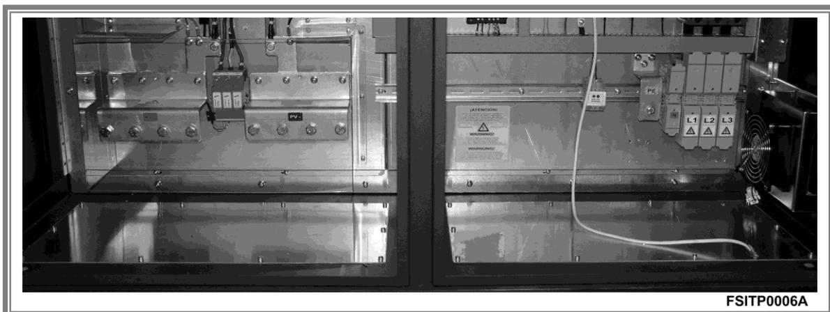
Figure 2.6 View of the base plates for cable routing and the FREESUN electrical connections
