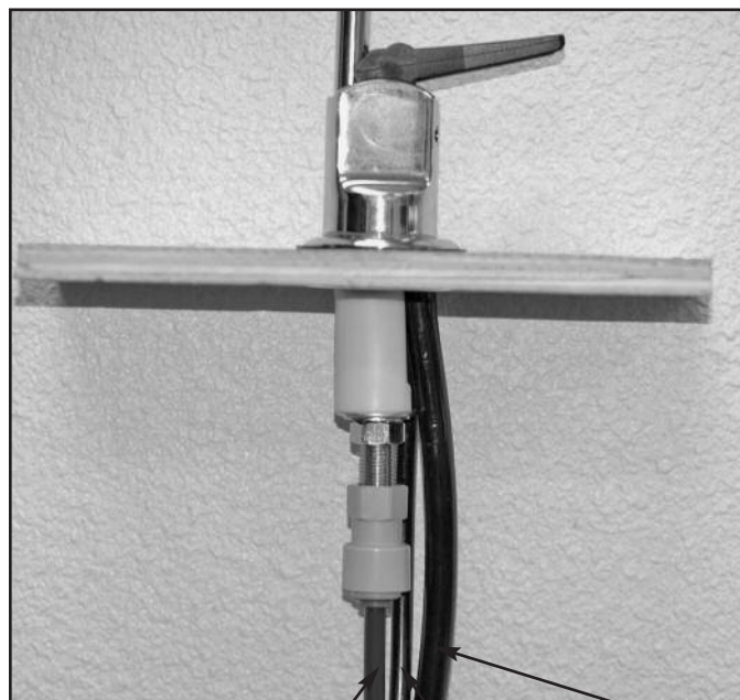
← Completed Air gap faucet installation
