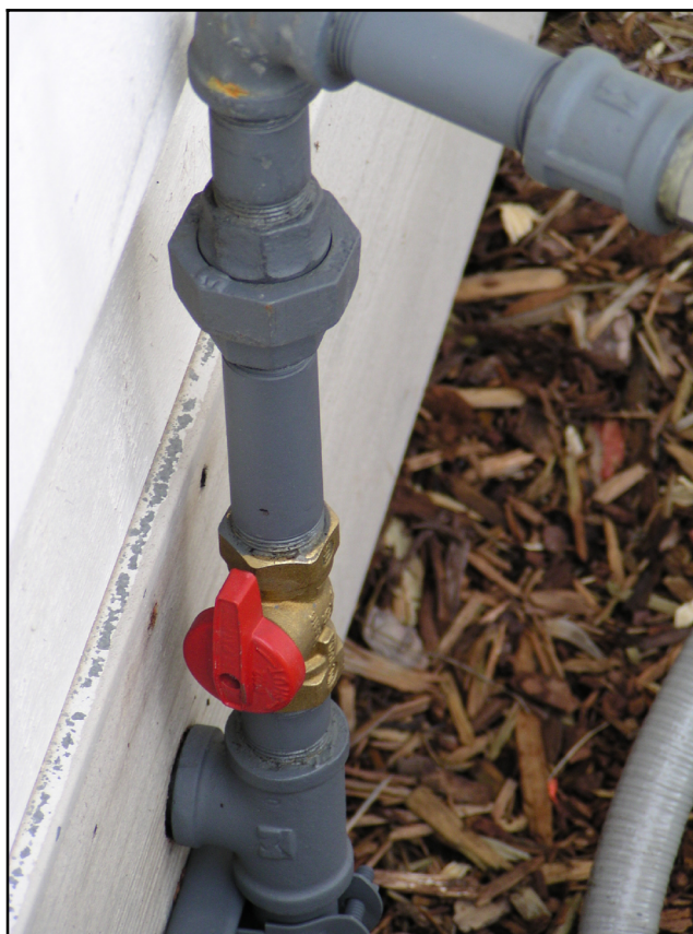
Figure 2-5 Manual Fuel Shutoff Valve (outdoor installation shown)
