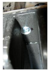
Running the fan 24/7 wears it out. A better choice is have it come on only when needed. This is done with a thermo switch; normally open, then closes at 100°F. For redundancy, two of these switches are mounted, in parallel. Use a good layer of heat sink compound under each switch.
