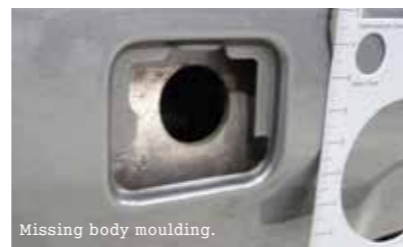
Examples shown are of unacceptable damage.
