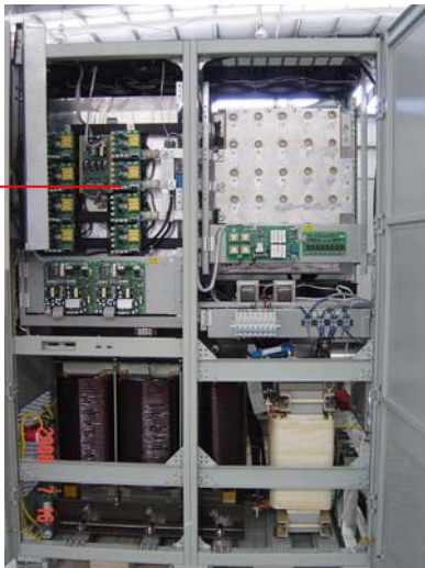
Picture 3-9 200~400KVA inverter module, rectifier module, bypass and output SCR module
