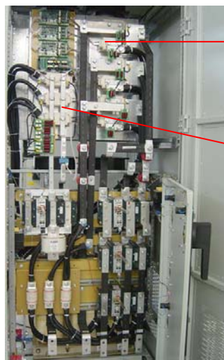
Picture 3-9 200~400KVA inverter module, rectifier module, bypass and output SCR module
