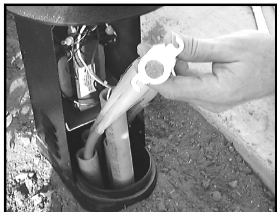
10. Inspect the cut, no lines or "puddles".
