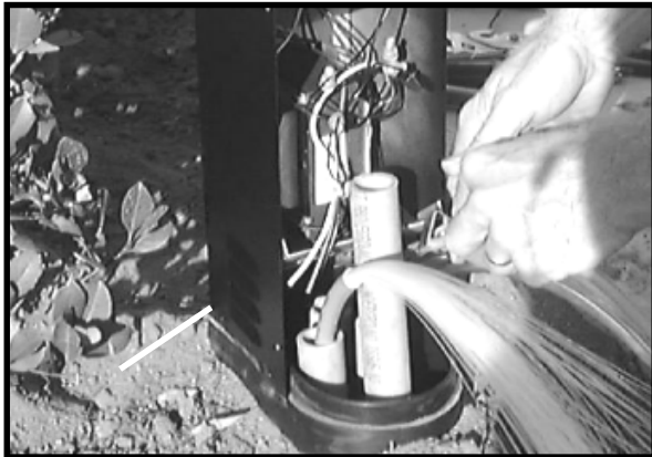
2. Strip jackets from 3 to 4 in. above the base.
