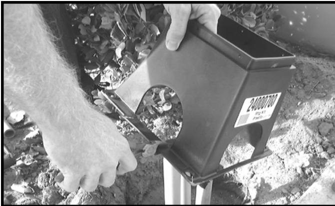
2. Cut subbase flanges as needed.
