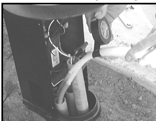
11. One wrap of the tape in the middle.
