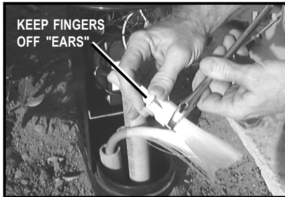
4. Securely tighten the ferrule assembly.
