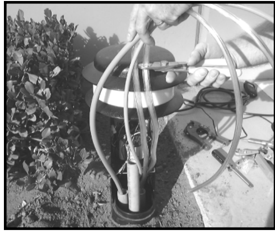
1. Cut all cables even with the generator top.
