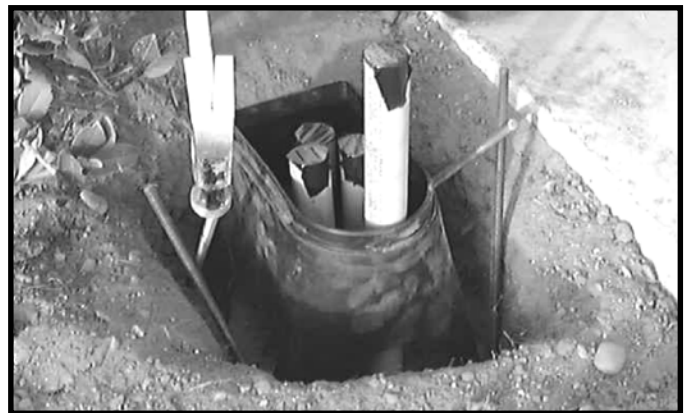
3. Drive 3/8 in. rebar at an angle in the corners.
