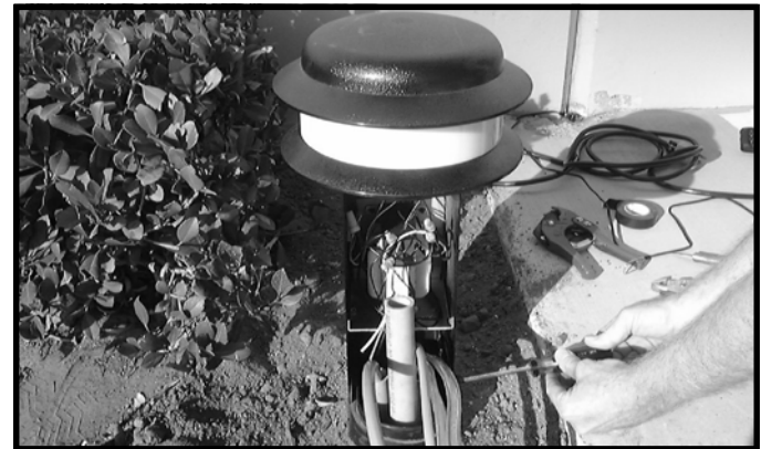
5. Secure the generator with the screws provided.
