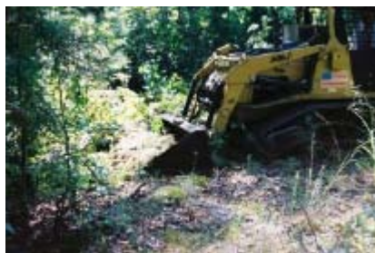
Picture 46 – Bucket moving debris
