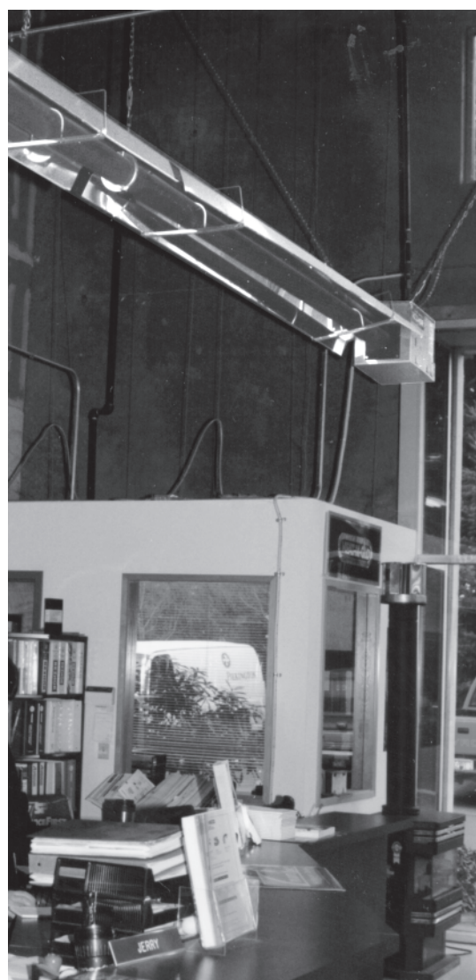
FIG. 31 - Service Counter Heating with Low Intensity Tubular Units
