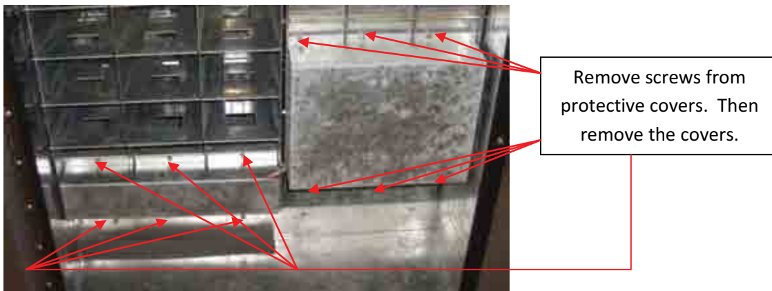
Figure 49 – Remove protective covers
