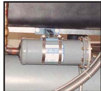
Typical filter-drier Figure 6.2D
