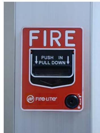
**Figure 27: Fire Alarm Pull Station**
