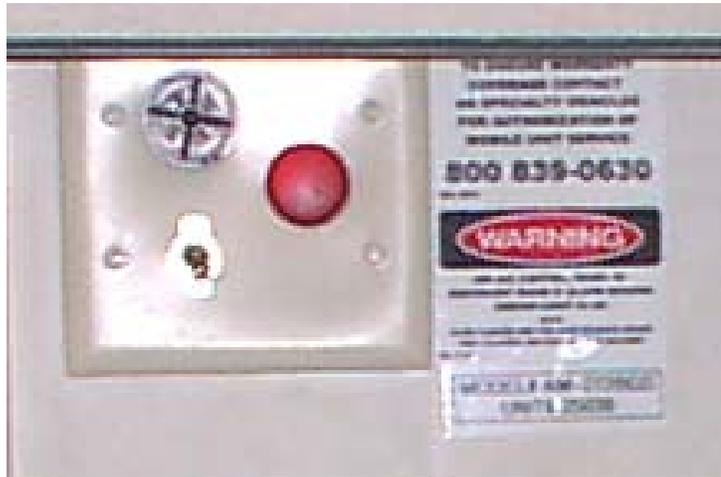
**Figure 45: A/C / Chiller Alarm Panel**
