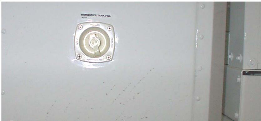
**Figure 41: Humidifier External Water Connection**
