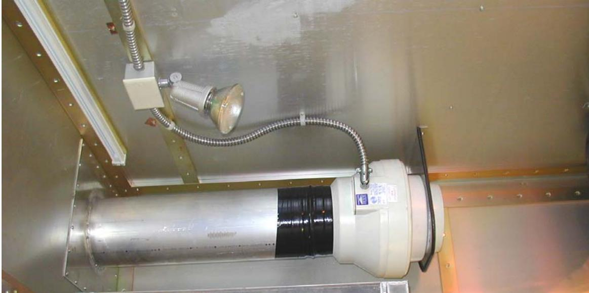
**Figure 14: Magnet Room Helium Gas Exhaust Fan**
