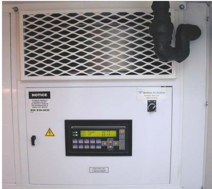
**Figure 44: A/C / Chiller Control Panel**
