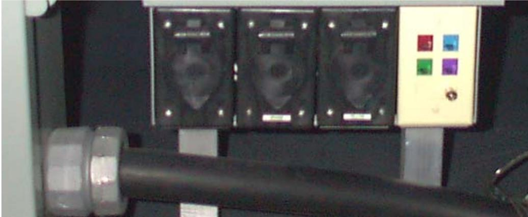
**Figure 16: Phone & Data Line Connections**
