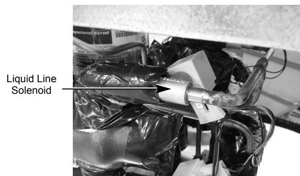
Figure 47. Liquid Line Solenoid (1 per barrel)
