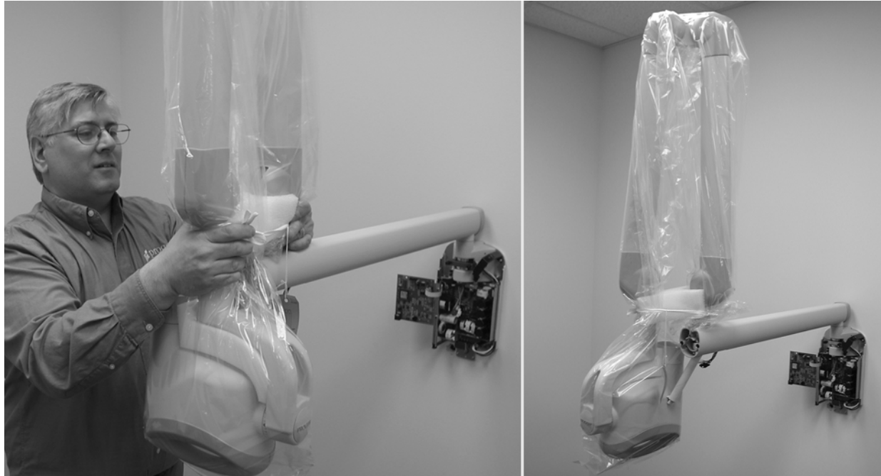
Figure 19 Installing the Articulating Arm and Tubehead Assembly
