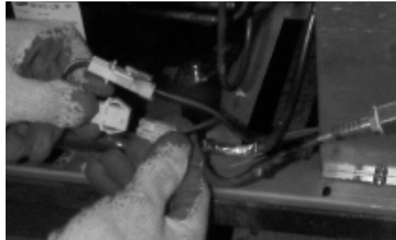
DISCONNECT THE CONNECTORS
