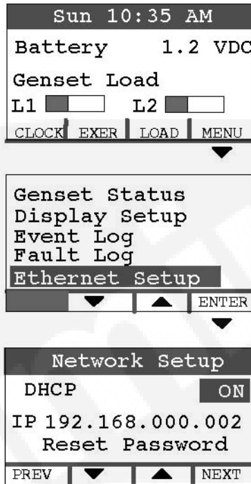
FIGURE 30. NETWORK SETUP SCREEN ON THE IN-HOME OPERATOR PANEL
