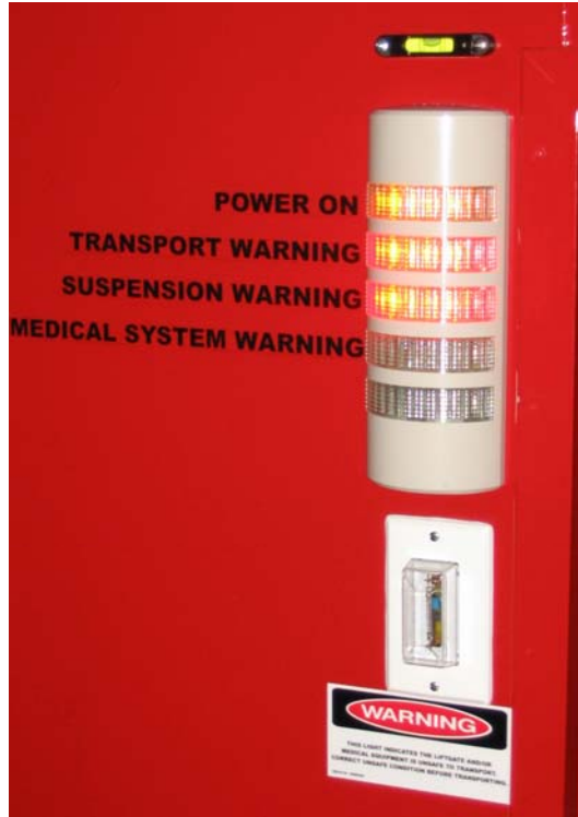
Transport Warning Lights
