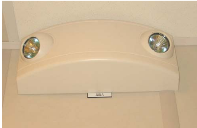
Figure 74: Emergency Dual Beam Lighting (Typical)
