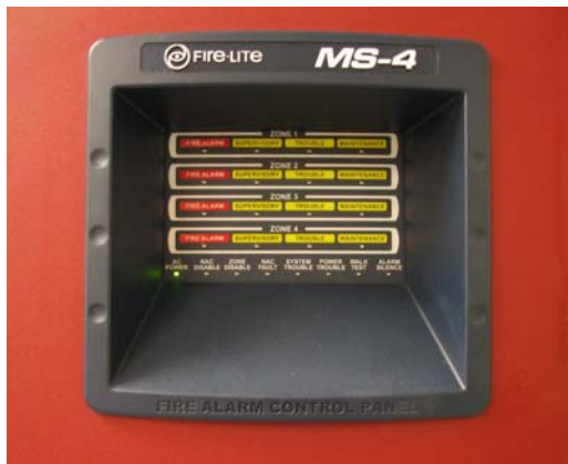
Figure 3: Fire Alarm Control Panel MS-4 (Four Zone)
