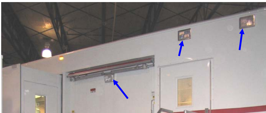
Figure 77: Staff Door Lighting
