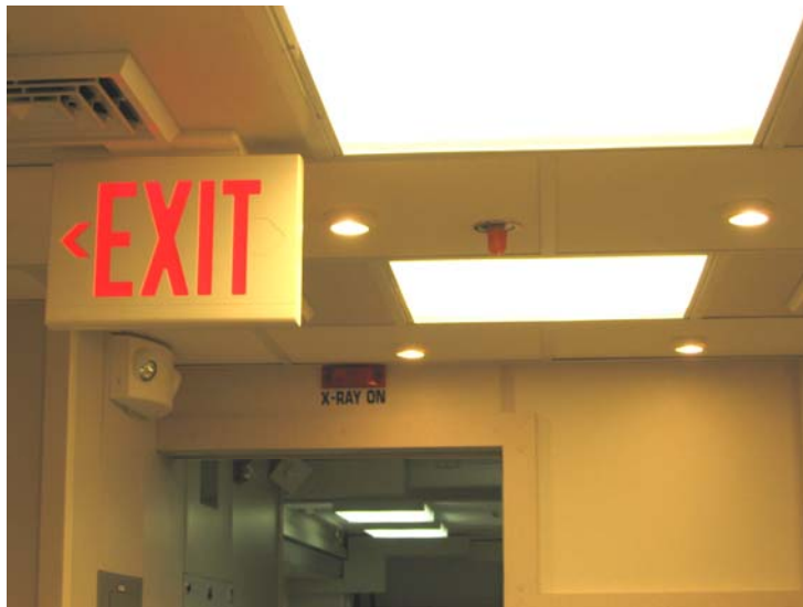
Figure 78: Control Room Lighting
