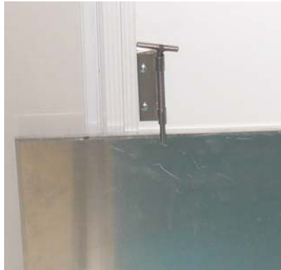
Figure 58: Patient Door Inner and Outer Floor Transition Plates Up and Locked
