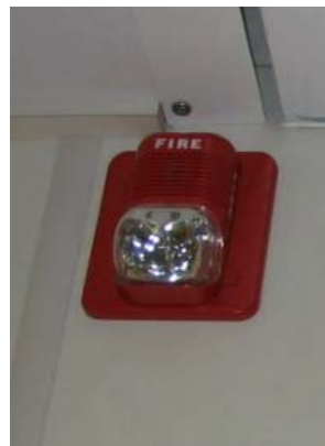
Figure 33: Fire Alarm Pull Station and Strobe lights
