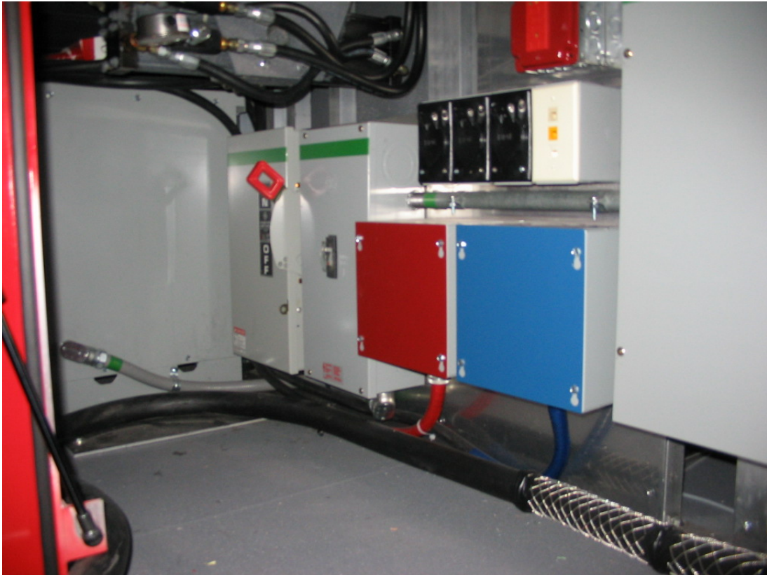
Figure 25: Phone and Data Line Connections (Typical)
