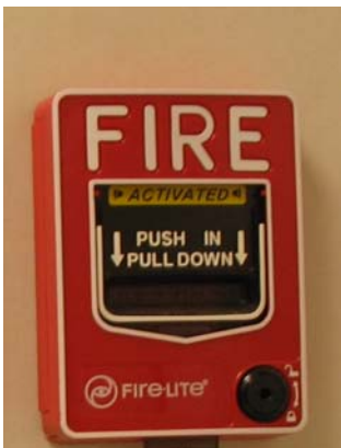
Figure 33: Fire Alarm Pull Station and Strobe lights
