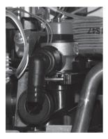
**Caution:** Do not under any circumstances manipulate the safety valve during the operation of the boiler. The safety valve furthermore may not be used for releasing water from the boiler or the heating system. The settling in the valve of detritus from the heating system is not covered by the warranty.
