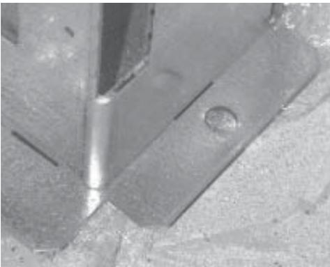
Loosen the two screws that hold the bracket to the support bar and rotate the unit to one side so you can access the mark for the floor hole. Drill a hole suitable for the 10mm (3/8 in) fixing hardware being used.
